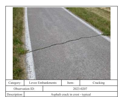
0207 - No User Rating (Site Visit) - Asphalt crack in crest - typical
